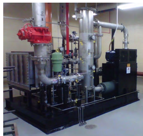
Figure 5-5 Representative Biogas Booster System
