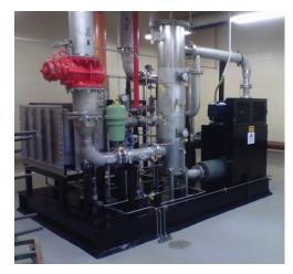
Figure 3-3 Representative Biogas Booster
